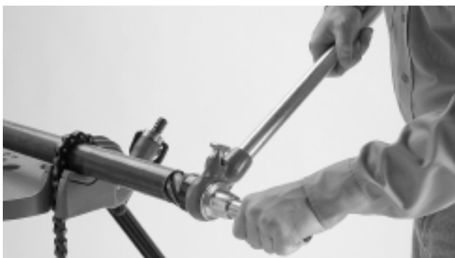
Figure 2 – Reaming End of Pipe
